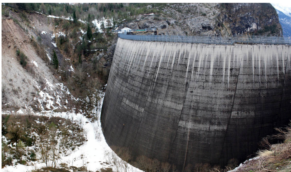
The Vajont Dam as seen from the Friulian side
